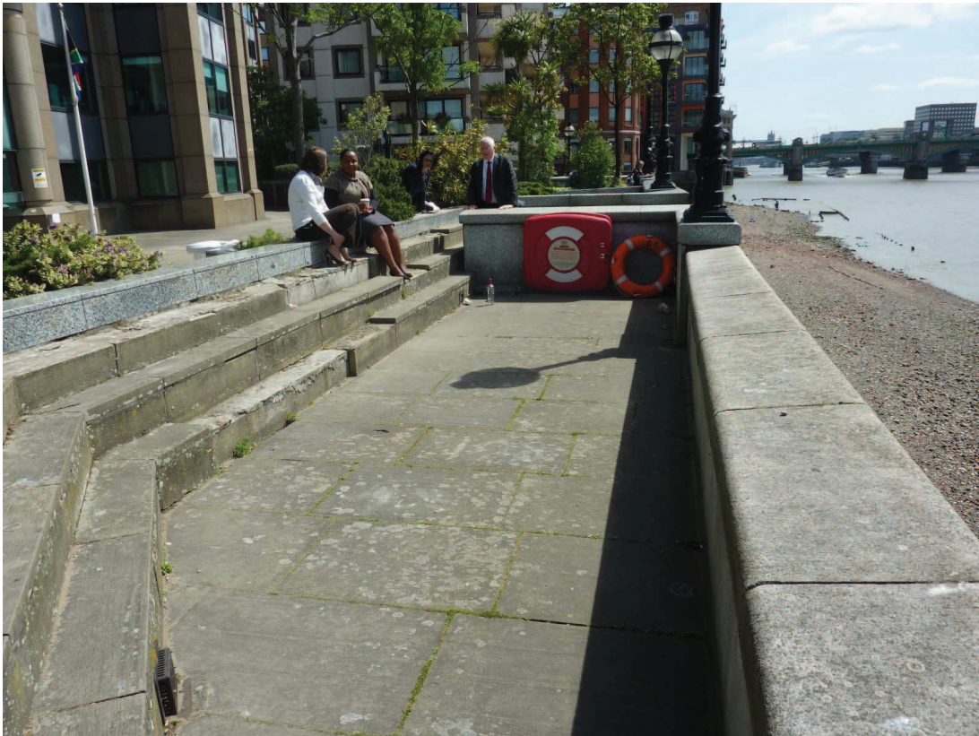
Existing Planter adjacent to the Riverside Wall
